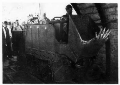
LZK-1-p ROCKER SHOVEL LOADER looks surprisingly like the Eimco 12-B Rocker Shovel which was the first loader of this type in the world. Note the interested spectators at this model mine somewhere in the Soviet Orbit.
